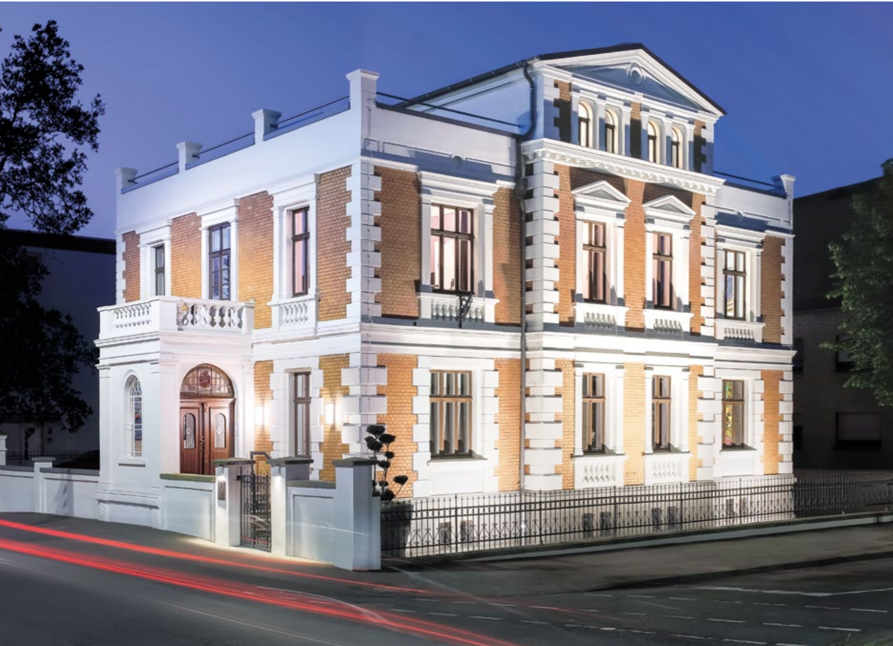
Kitzig Design Studios was founded in Lippstadt. The office is located in a renovated city villa.
